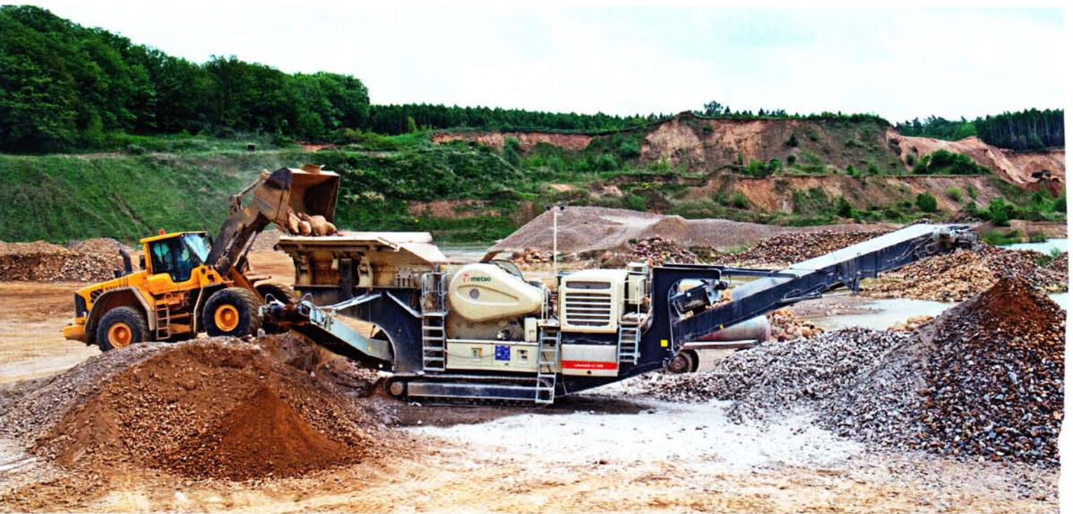
1 Neueste raupenmobile Brechanlage Lokotrack LT120E von Metso • Latest track-mounted Lokotrack LT120E crusher from Metso
